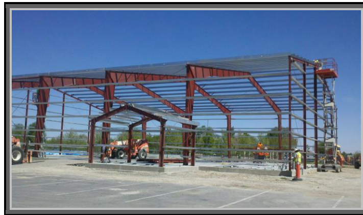
Multipurpose Recreational Facility: Fallon Nevada
